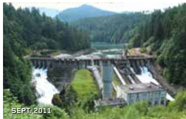
LEFT The Elwha Dam demolition.
