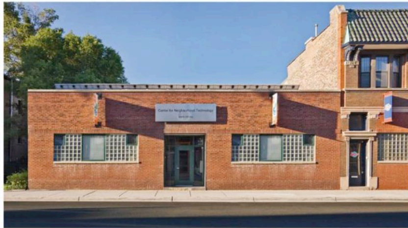
Above Chicago's new Center for Neighborhood Technology is a LEED Platinum certified renovation of its 1920s headquarters, a former textile factory.
